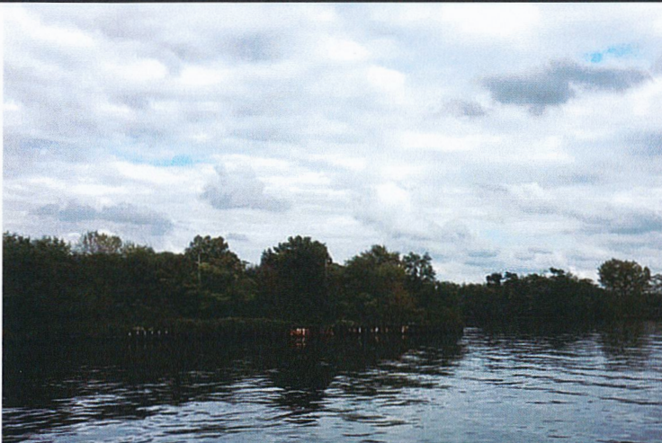
Photograph No. 7 – View of sheet piling water's edge
